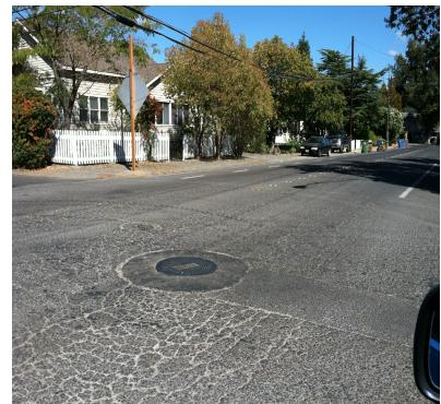
The streets will be ground up and mixed with cement to create a hard base before paved with a new asphalt concrete surface. The full depth road reclamation will reduce costs by recycling some of the existing road materials and reduce green house gas emissions by reducing trucking between the batch plant and Project. Madison Street is one of the few truck routes across the Napa Valley and has been designed for the additional traffic loads.
