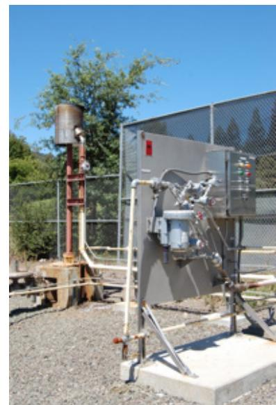
The methane recapture program, completed in 2012, uses digester gas produced during wastewater treatment to run the treatment plant. About 61 percent of the digester gas is used for fuel and the rest is flared off.
